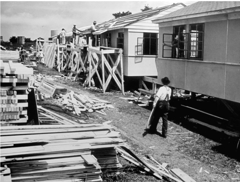
Figure 8. TVA Assembly Line for the Production of “Truckable” Homes (Source: TVA Archive, National Archives Building, Atlanta, GA, Collection RG 142, Box 17)
