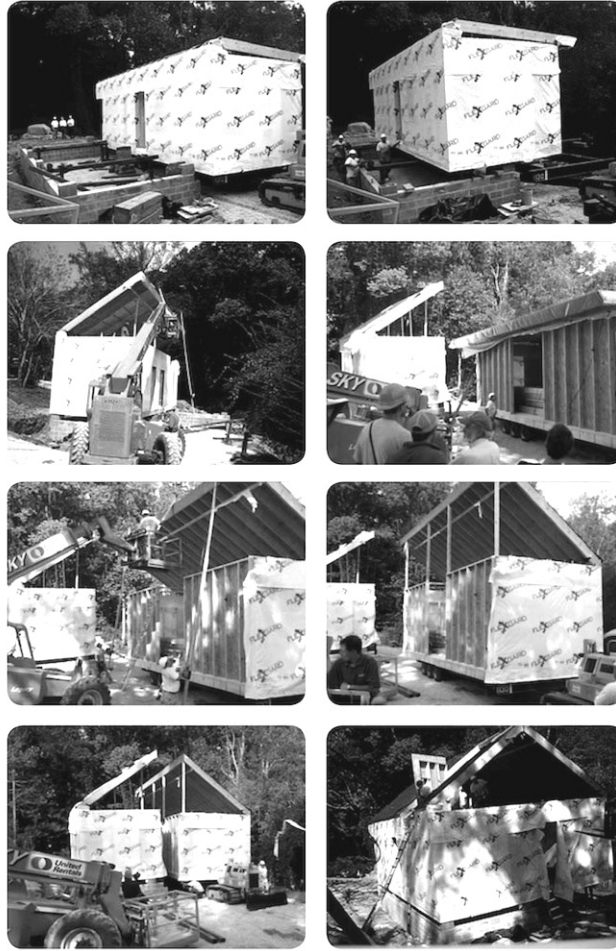
Figure 12. Assembly and Delivery of Prefabricated Components of the New Norris House (Photographs by Samuel A. Mortimer)
